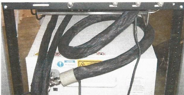
Above: System line looped and installed
