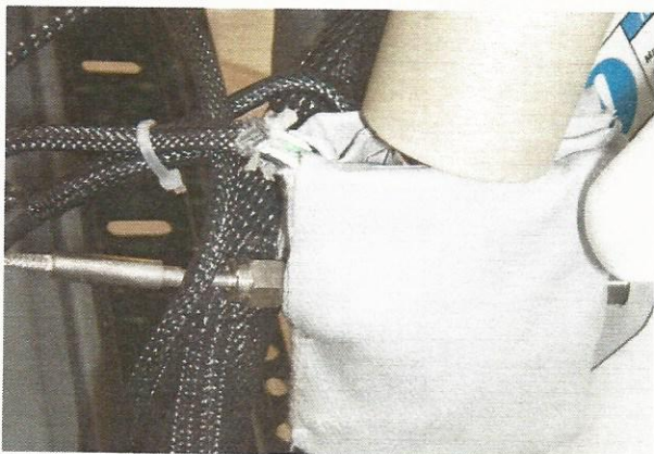
Above: Junction slave heater and temperature probe installed
